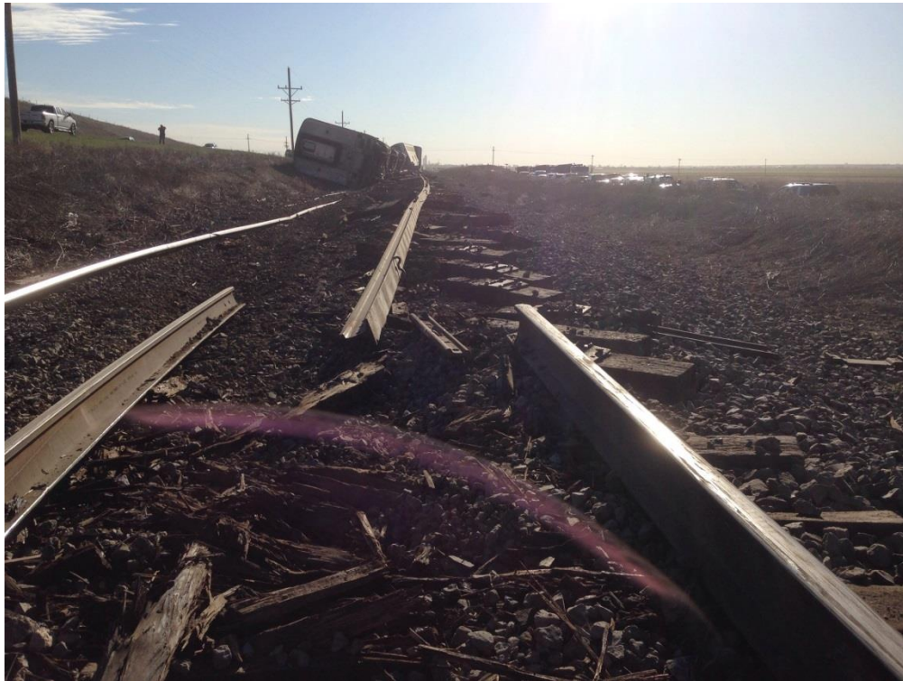
Figure 4. A view looking east at the derailed equipment cars and damaged track.
