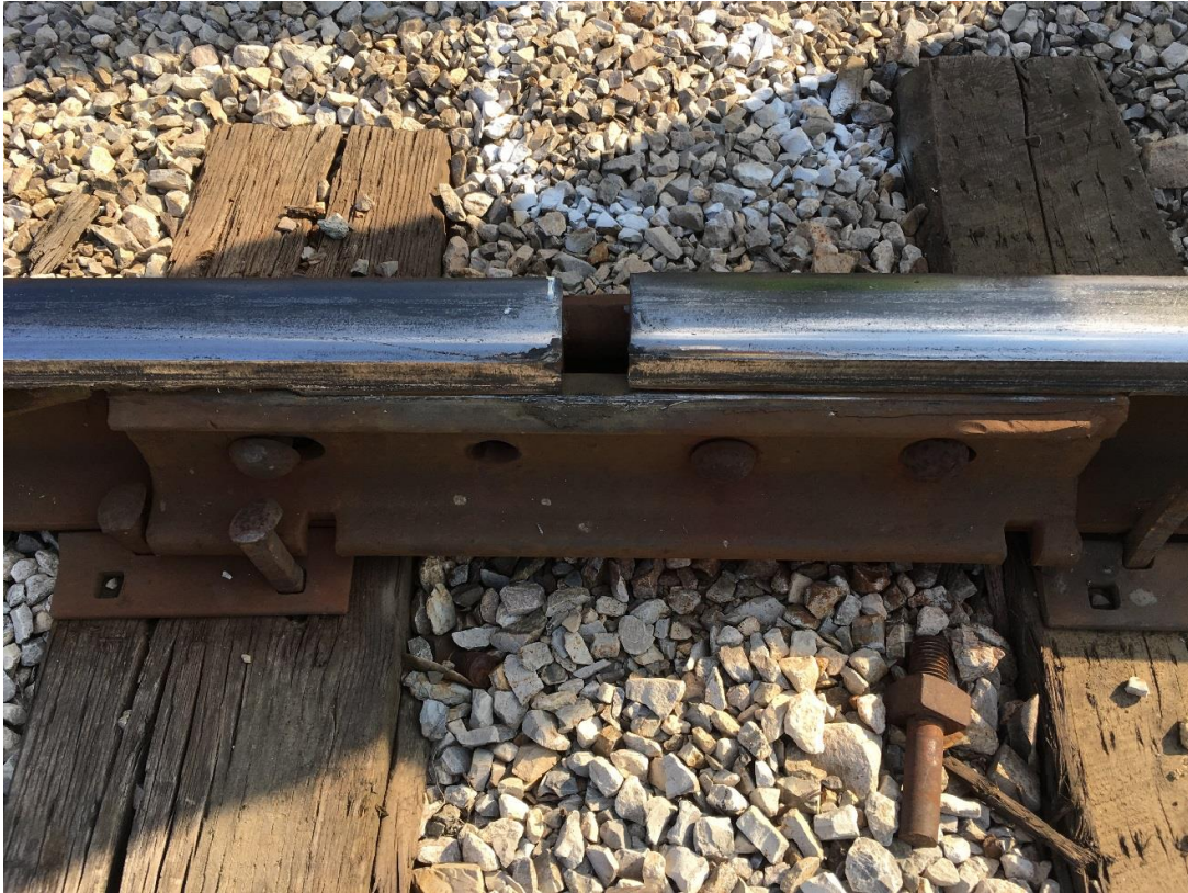
Figure 3. Rail Joint where wheel flange marks originated (POD).
