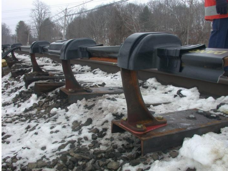
Figure 4-Northward view of the third rail assembly that replaced the damaged sections.
