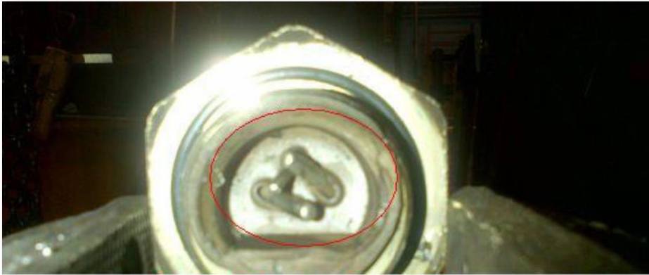
Pins twisted, caused by a seized jam nut (can happen when installing or removing cables)
