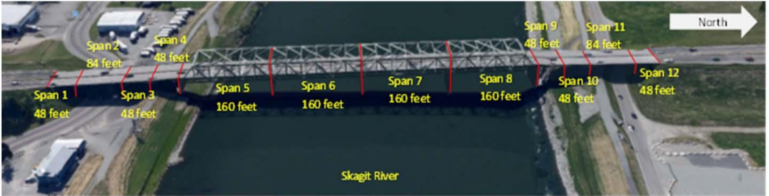
Figure 2: Bridge span orientation (Google Earth).
