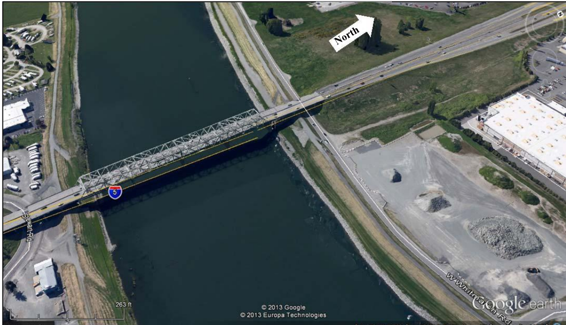
Figure 1: Aerial view of bridge as captured by Google Earth in 2011.
