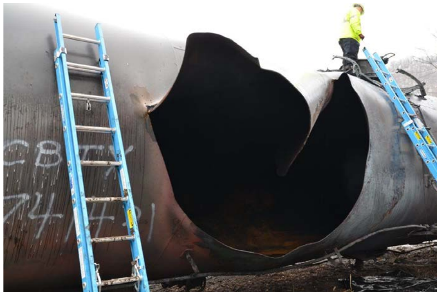
Figure 5: Tank car CBTX 741431 thermal shell tear.
