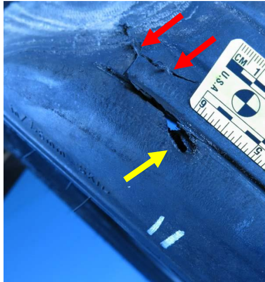
Figure 16. Hole in tread. (See yellow arrow from left) Material displaced outward is above the hole. (See red arrows from right) As installed, the tire would roll toward the camera.
