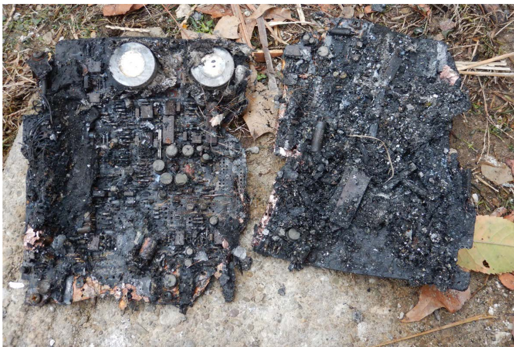
Figure 14 – Pieces of a Suspected DEEC Board at Accident Site.
