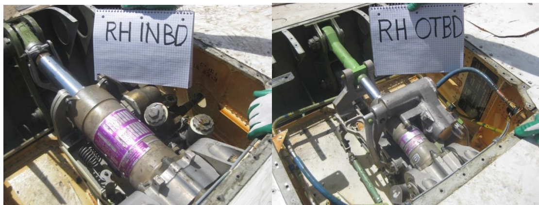
Figure 5 - Right Inboard PCU (Left) and Right Outboard PCU (Right) after the access panels were removed.
