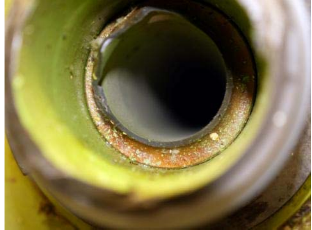
Figure 28: End view of fractured safety rod
