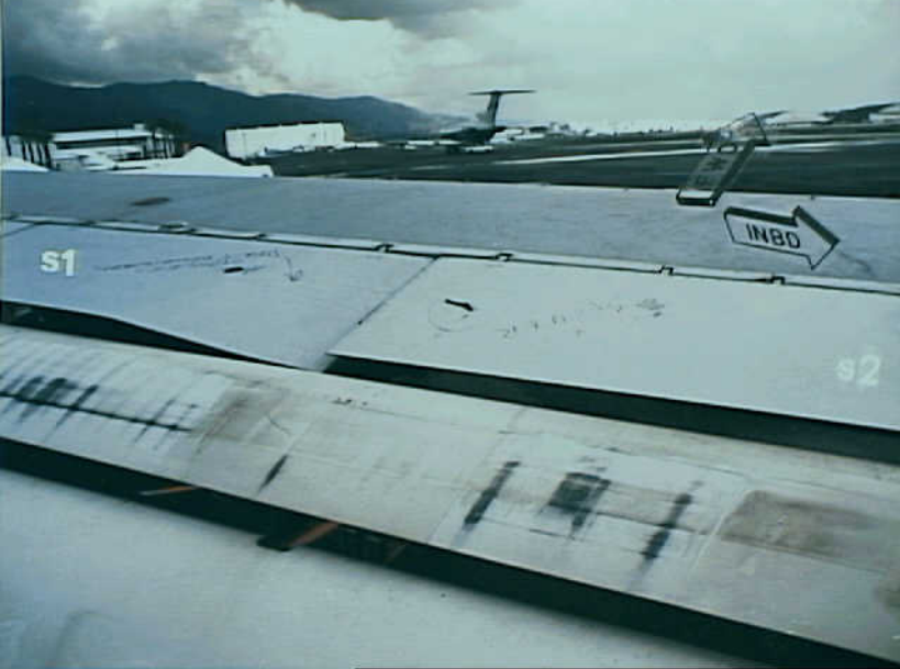
Systems 9 - Photo 9. View looking forward of spoiler 1. Note damage to inboard trailing edge. There was no damage to the leading edge of the flap panel.
