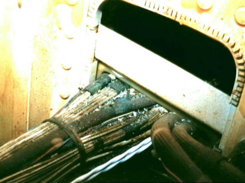
Systems 9 - Photo 52. (Feb. 21-25, 1998) B-747 station 400 opening and wires in raceway clamp. Visible are metal shavings, yellow/brown corrosion-inhibitor, bright white wires routed with darkened wires.
