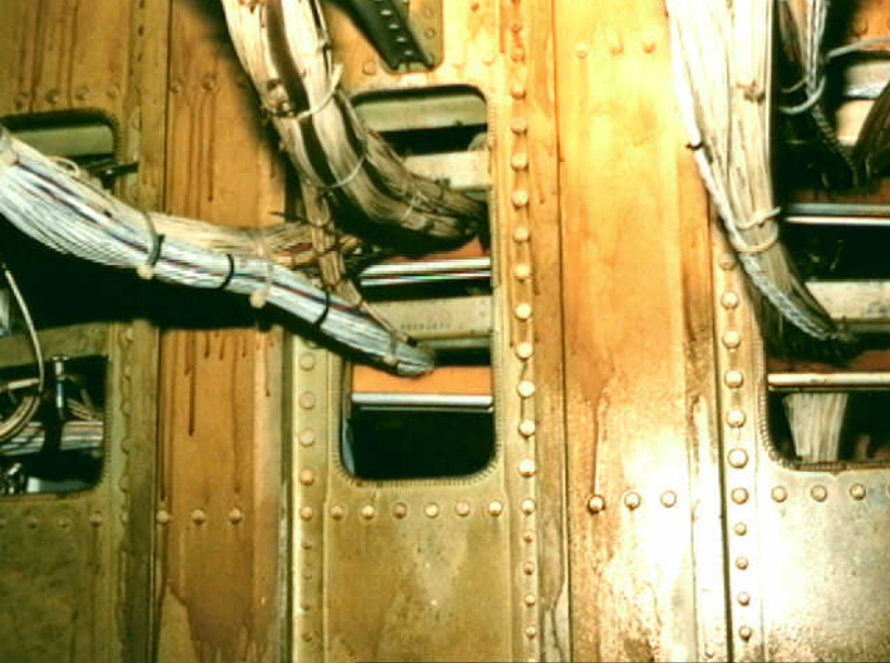
Systems 9 - Photo 50. (Feb. 21-25, 1998) B-747 station 400 (right), viewed aft from the right of the nose landing gear. Wires for #4 fuel flow and CWT FQIS signal are in the center opening. Visible are corrosion-inhibitor (brown drips) and blue stains.
