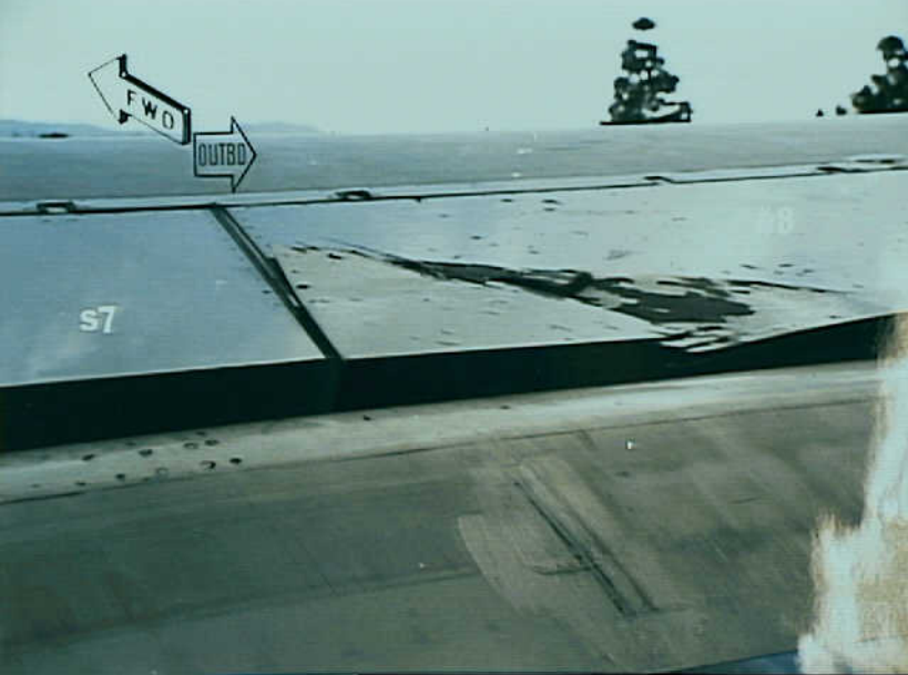
Systems 9 - Photo 10. View looking inboard of spoiler 8. Note damage to inboard trailing edge. There was no damage to the leading edge of the flap panel.
