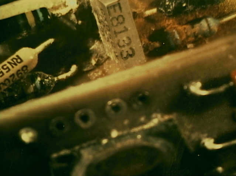
Systems 9 - Fuel Quantity Indicators - Photo 6. Totalizer component date code E8133 is visible.
