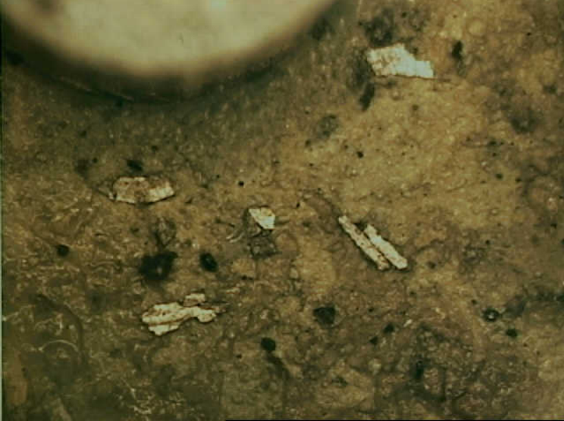
Systems 9 - Fuel Quantity Indication System - Photo 48. Metal shavings adhered to the STA 940 floorbeam lower cap at LBL 65, typical of shavings from LBL 40-70. The large round shape is the bucked end of a rivet.
