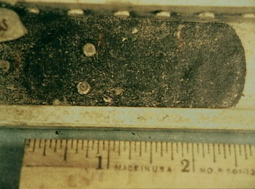
Systems 9 - Fuel Quantity Indication System - Photo 11. Sealant with drill shavings at bottom of STA 920 floorbeam. (Digital image)
