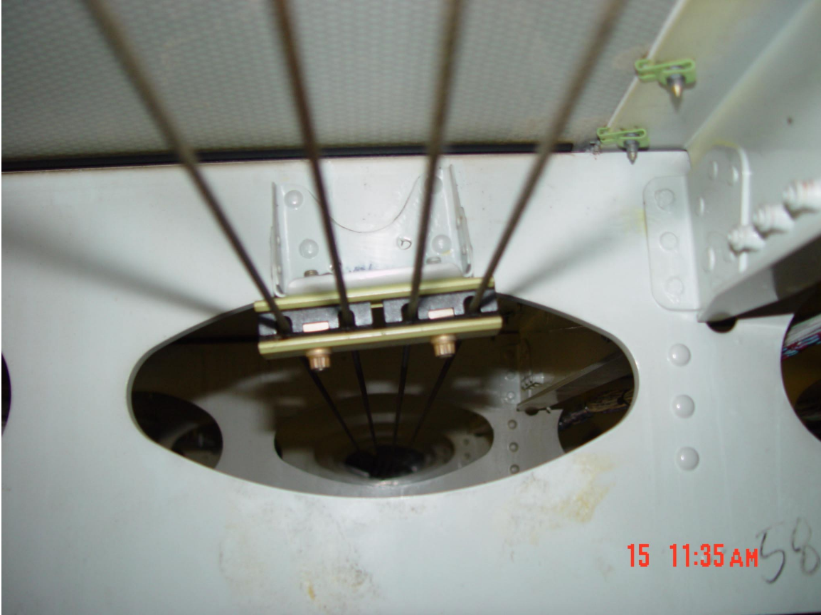
Figure 53. Frame C58 looking aft.
