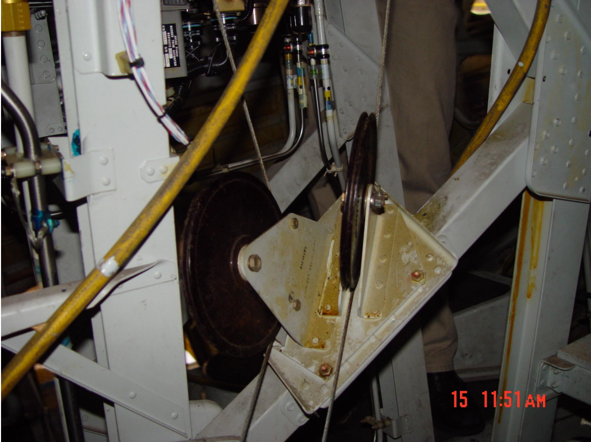
Figure 61. Yaw control cables and pulleys at rudder frame assembly.
