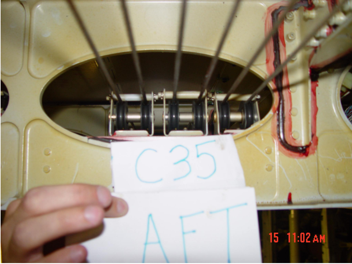
Figure 39. Frame C35 looking aft.
