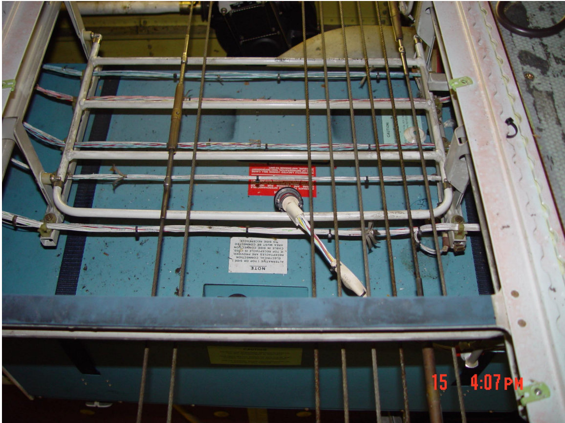
Figure 42. Frames C38.2 through C40 looking aft and down.
