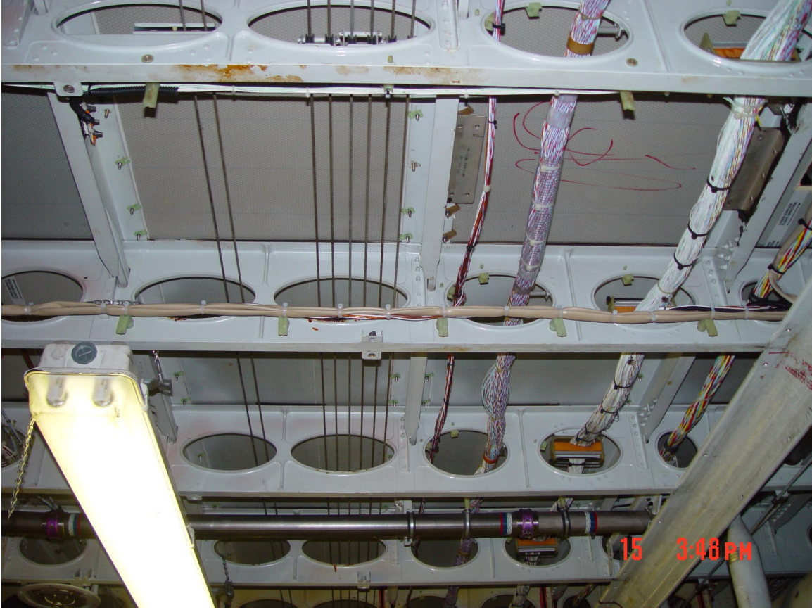
Figure 36. Frames C21 through C24 looking aft.
