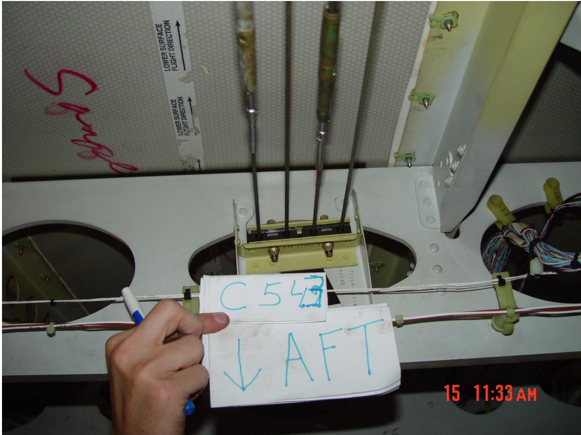
Figure 51. Frame C54.3 looking aft and up.
