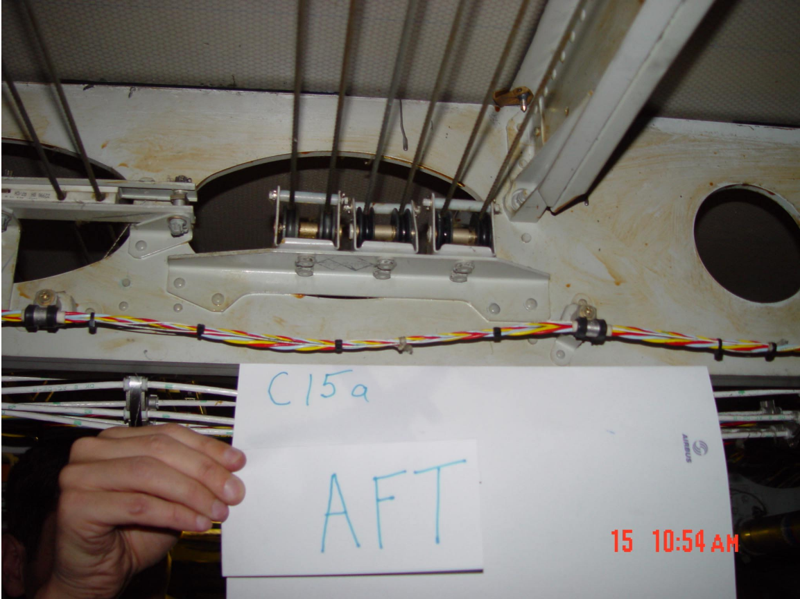
Figure 33. Frame C15a looking aft.
