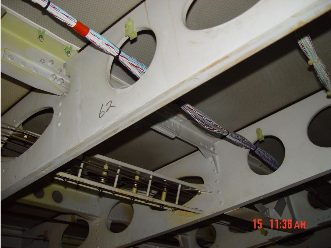
Figure 54. Pulleys between frames C62 and C63 looking up, aft and inboard.
