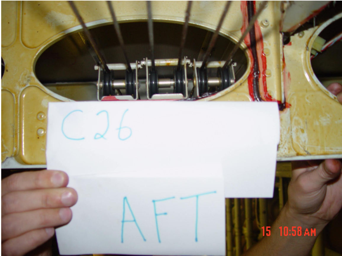
Figure 37. Frame C26 looking aft.
