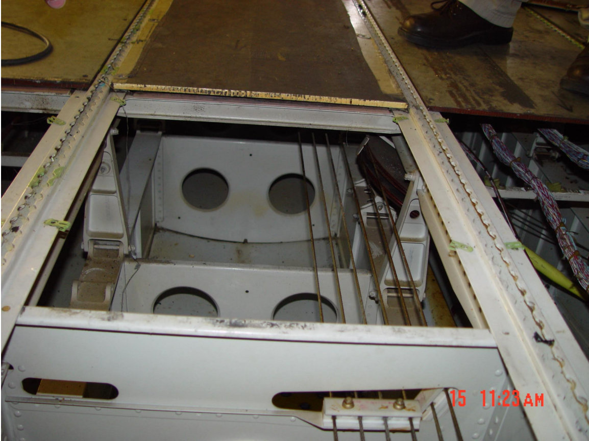
Figure 45. Frames C46 and roll control cable pulley looking aft and down.
