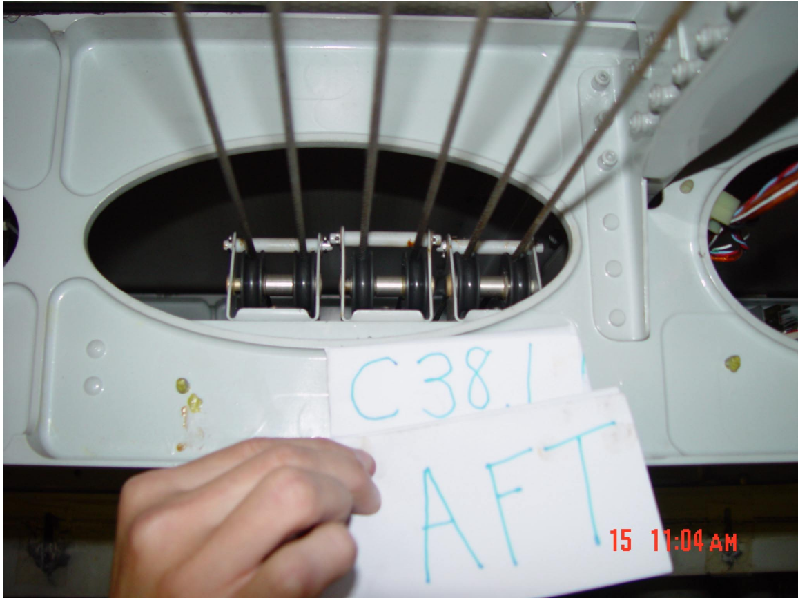
Figure 40. Frame 38.1 looking aft.
