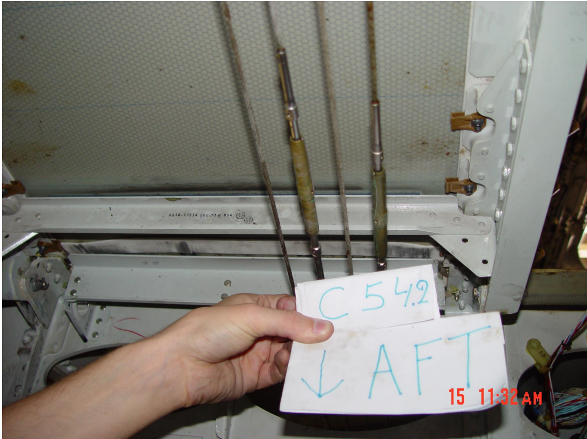
Figure 50. Frame C54.2 looking aft and up.
