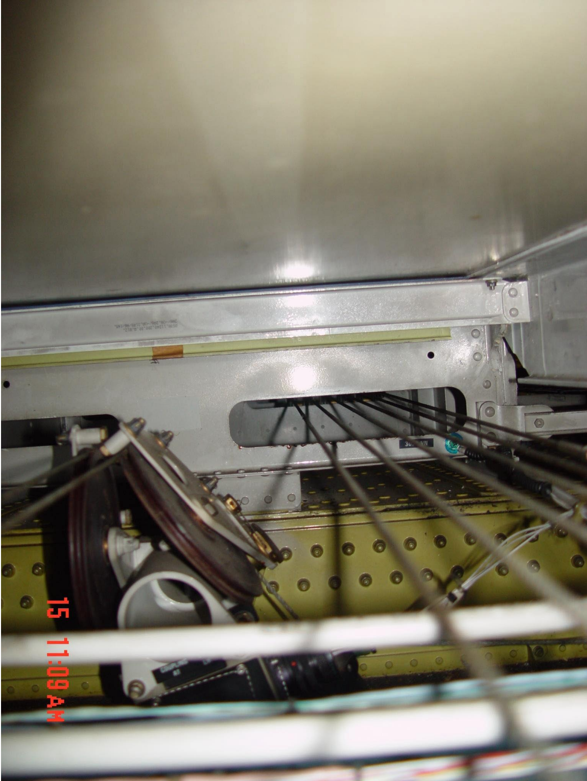
Figure 41. Frame 38.2 looking aft.
