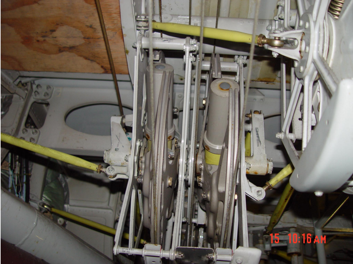
Figure 29. Roll (ailerons) and yaw (rudder) cable tension regulators, left to right respectively, looking forward.
