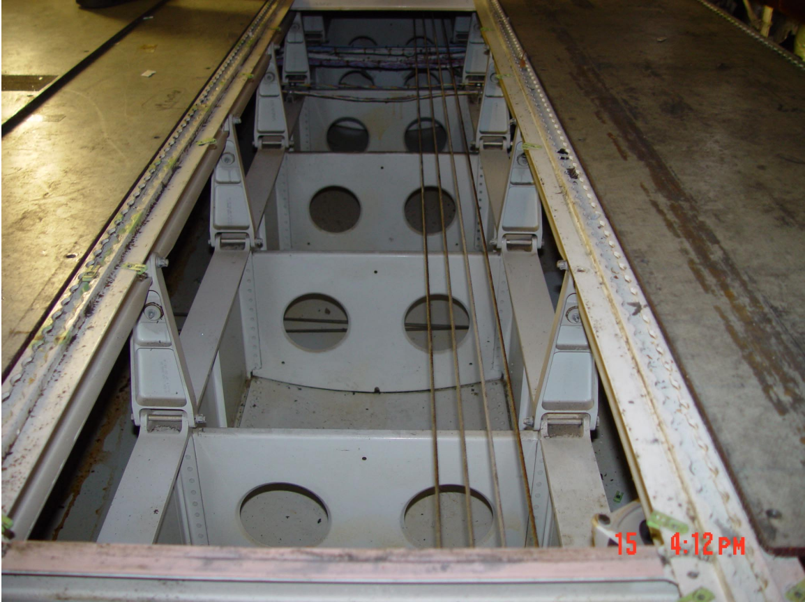
Figure 48. Frames C47 through C50 looking aft and down.
