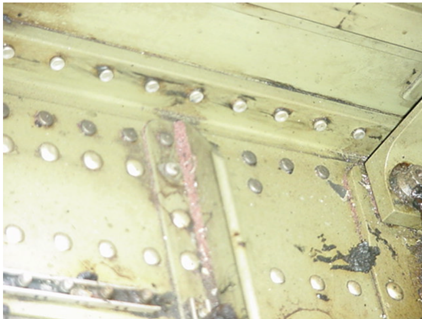
18. View of interior of the vertical stabilizer of a Hawaiian Airlines DC-9. This view shows the area just beneath the jackscrew assembly. Note pink granular material.
