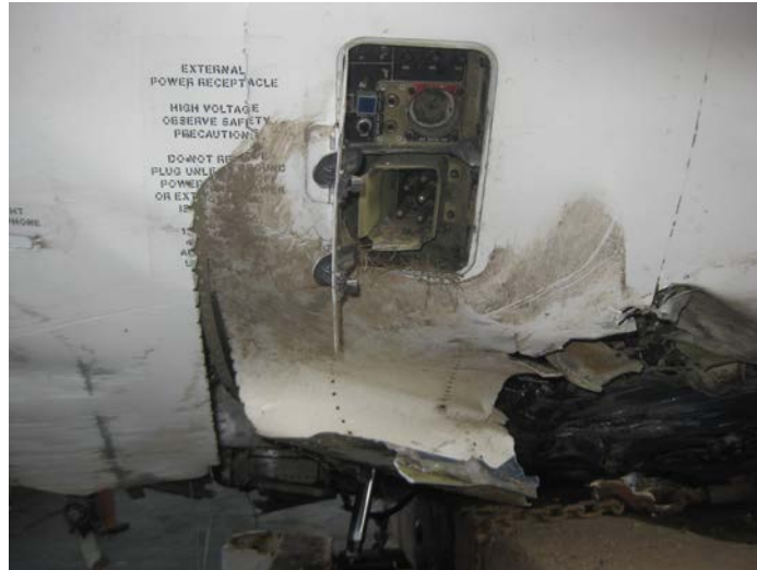
Figure 3 - Damage to area around the External Power Receptacle.
