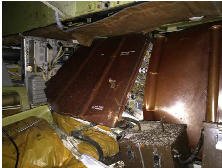
Figure 2 - Damage to Electronics Compartment, including Station 110 Relay Panel Cover.
