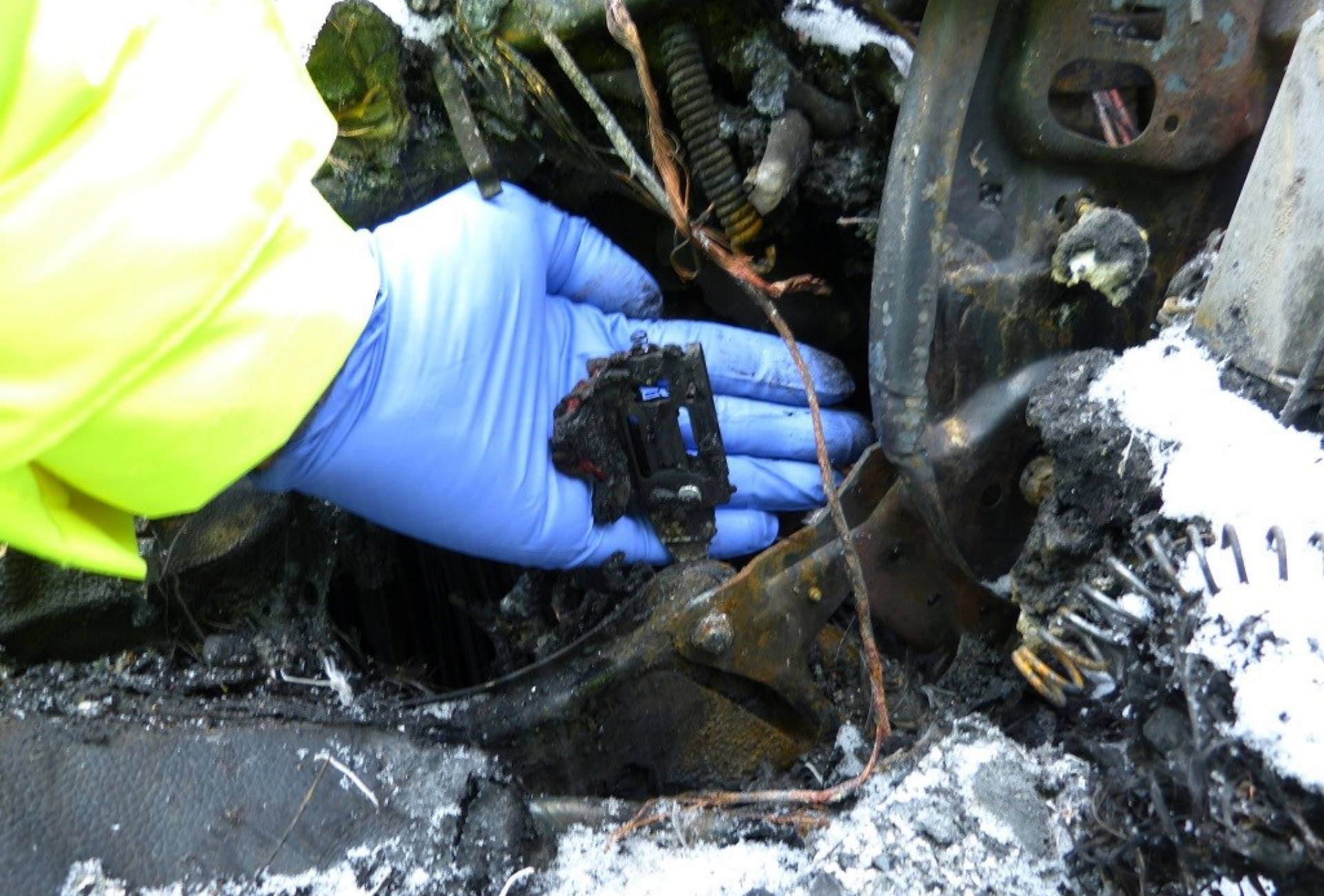
A detailed portion of the lower aft portion of the driver seat is visible. The driver seat belt buckle is visible, with severe fire damage having melted away most of the non-metal parts.
