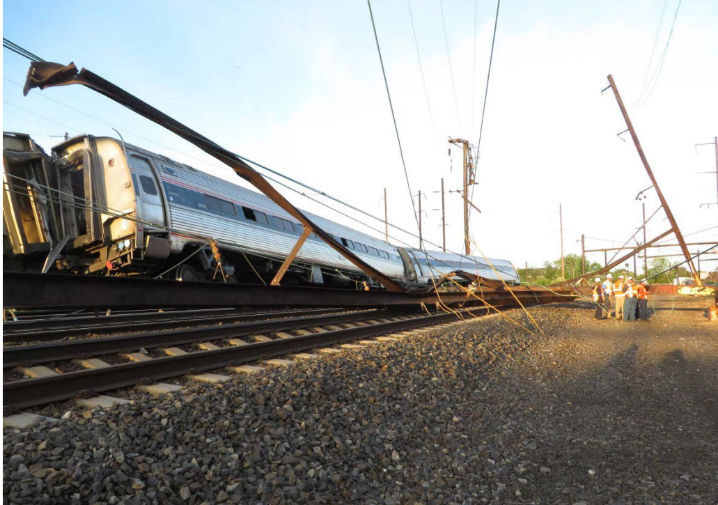
Figure 3. A view of the accident site showing the damage to the catenary system.
