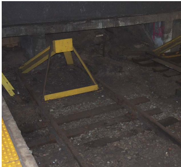
Figure 2- A bumping post on an adjacent track
