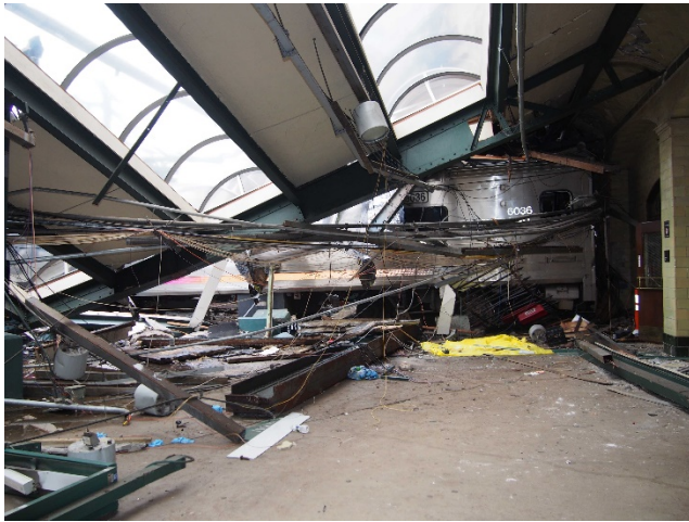
Figure 4- A view of the right side of the cab car
