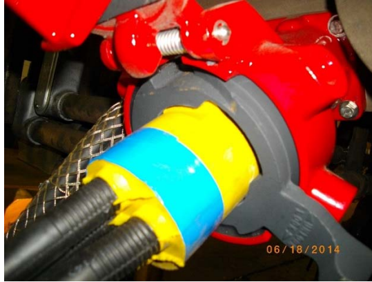
Photo – 480V Trainline Plug and Receptacle
