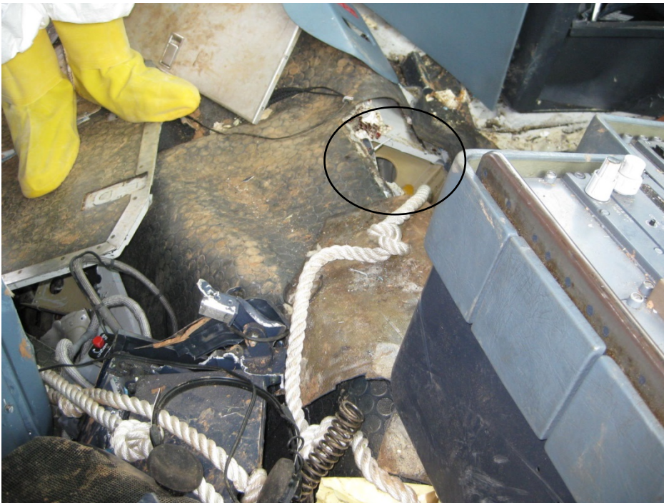
Photo 3. Buckling of flight deck floor, oval denotes original position of captain's seat base.
