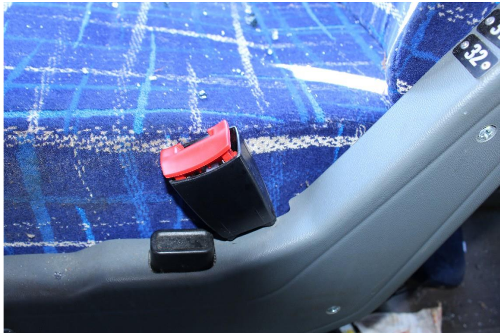
Photo #12: Defective aisle seatbelt buckle on motorcoach
