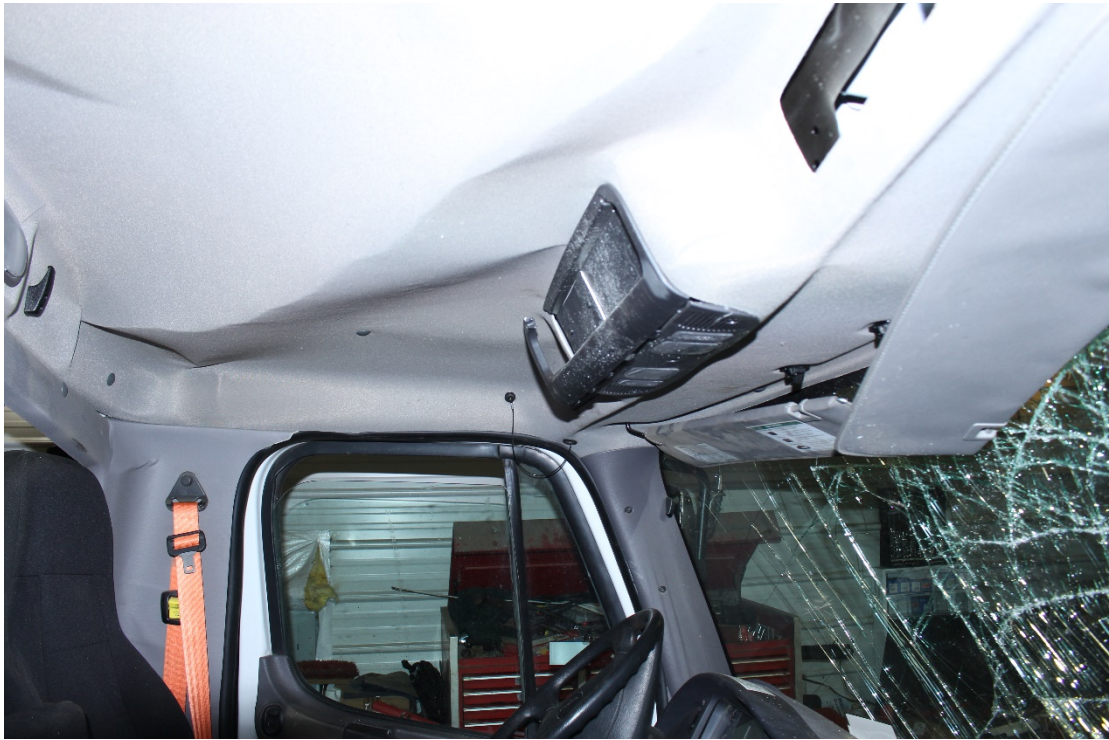
Photo #10: Interior view of trash truck cab showing close-up of roof deformation
