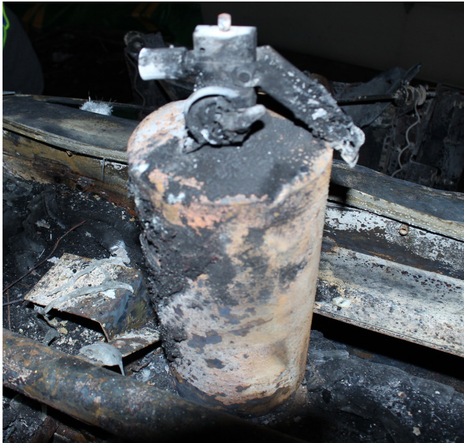
Photo #11: Close-up of fire damaged extinguisher
