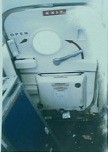
Survival Factors 6 - Photo 13. Fuselage damage, left side, with commingled approach light structure.
