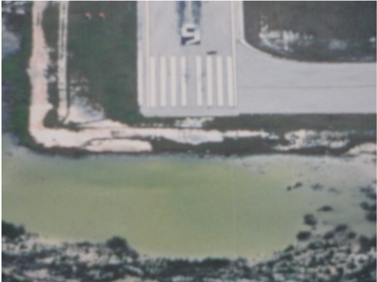
Photo 23: West end of EYW runway 9/27 before RSA improvements.
