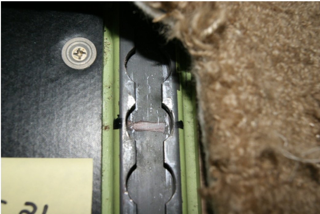
Photo 14: Seat L/H #2 forward inboard seat track.
