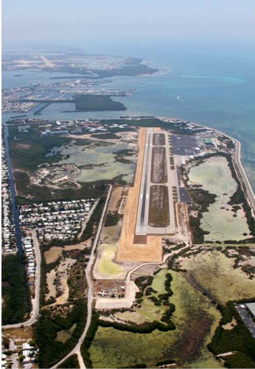
Photo 22: Aerial view of completed RSA reconfiguration.
