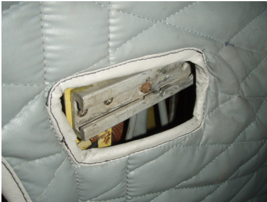
9. View of a section of seat track attached to the cabin sidewall where the single pin hold down fittings lock the side of the seat into the cabin sidewall.
