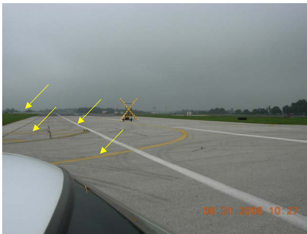
Photo 34. Runway 26 with the runway 4/22 intersection sign, lead-off line, white edge line, and yellow shoulder markings
