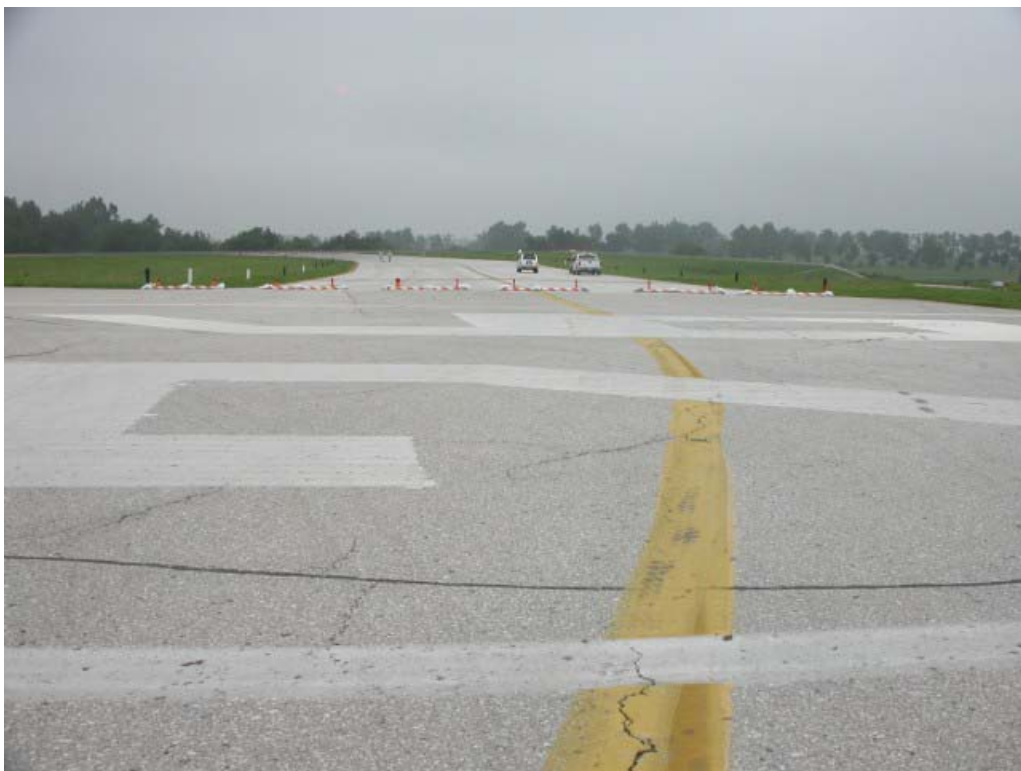
Photo 30. Old T/W A with lead-in line and low-profile lighted barricades
