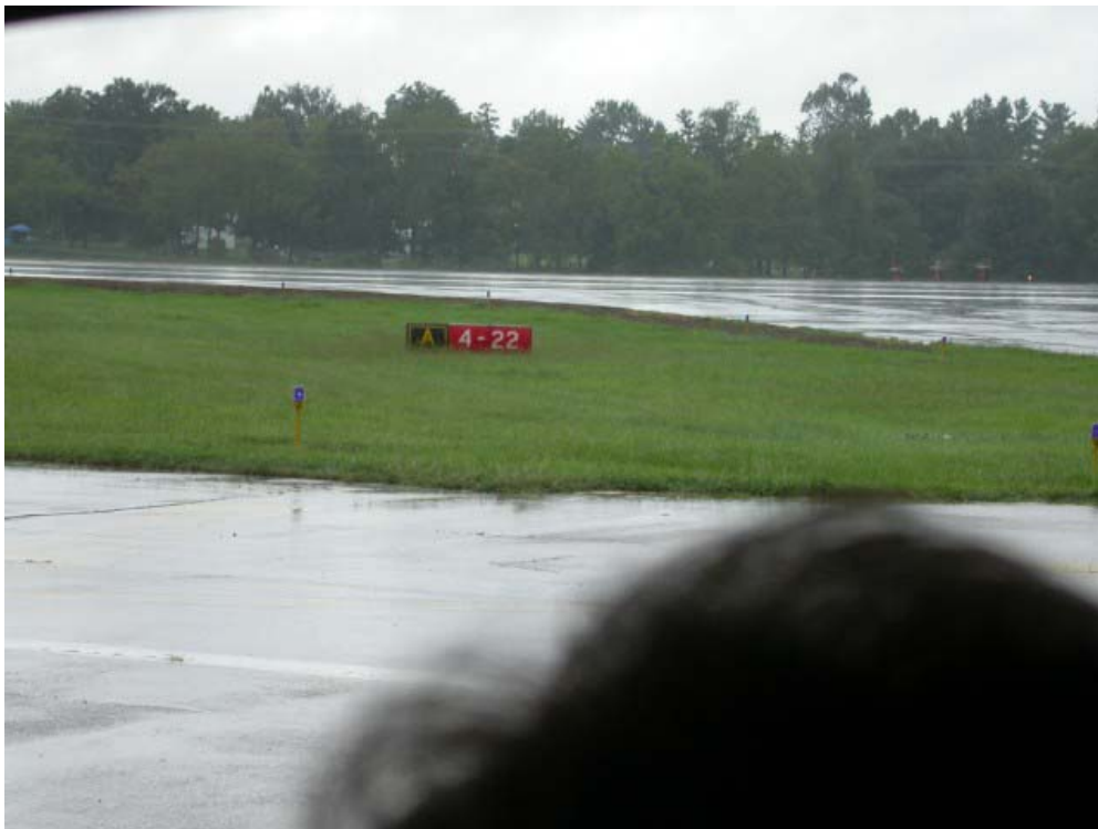
Photo 32. T/W A holding position sign for runway 22 as viewed from the centerline of runway 26
