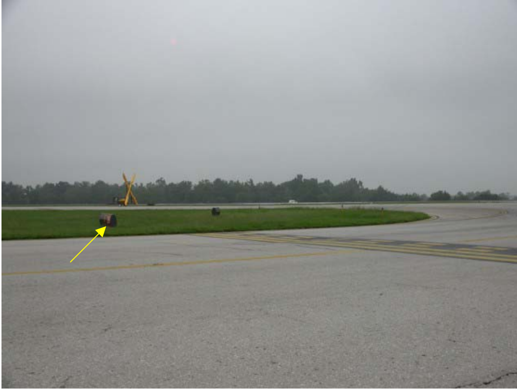
Photo 27. Location of T/W A holding position sign for runway 26
