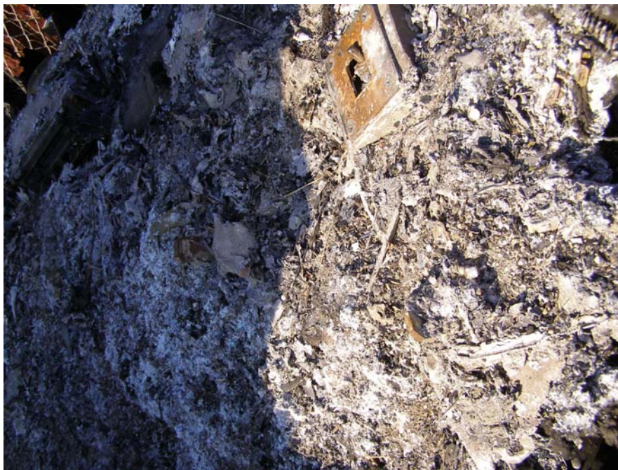
Photograph 10: MED components fused together in molten metal (Lancaster, TX).
