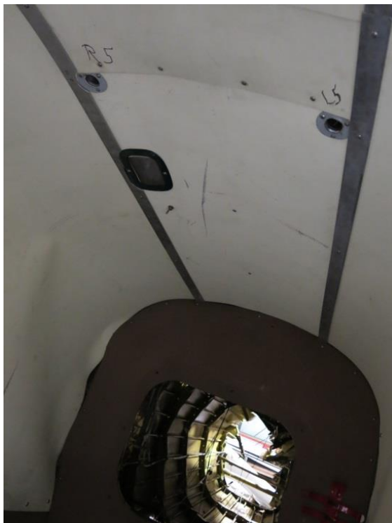
Photograph 38 –L5 and R5 ceiling attachment point.
