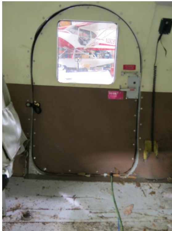
Photograph 43 – Photograph of the interior single entry door.
