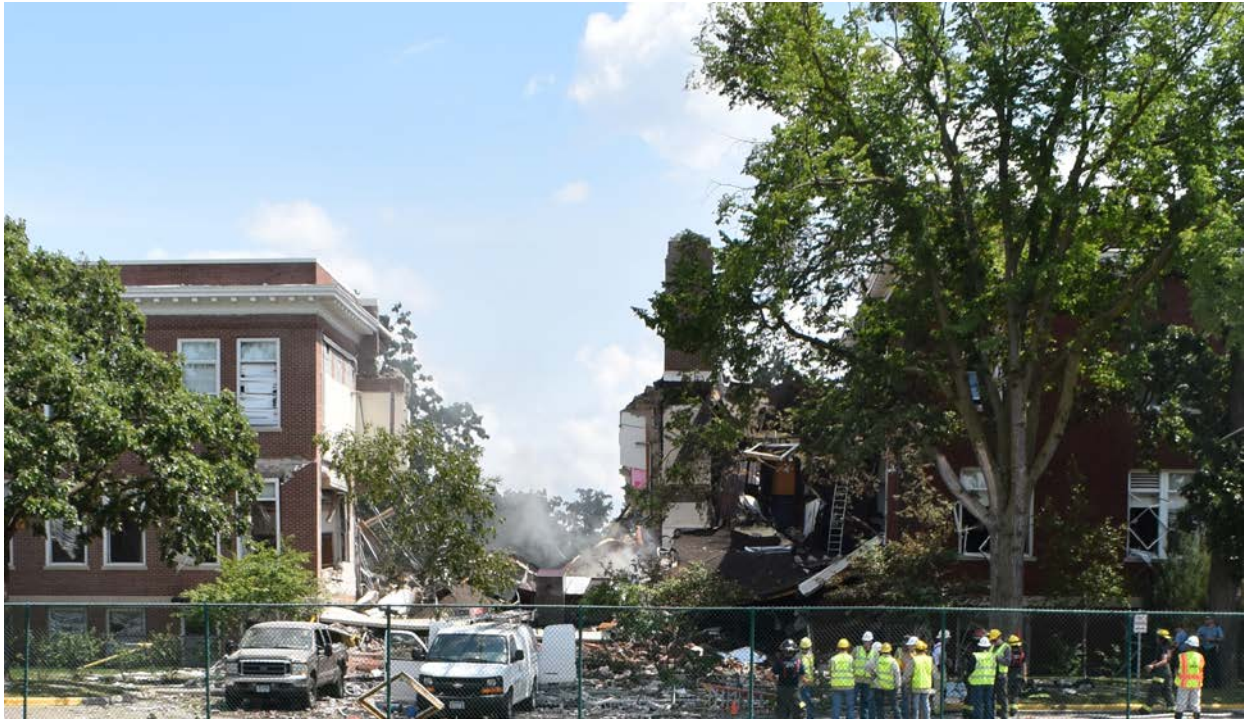
Figure 2. Photo of the accident site taken after the building explosion with several gas company personnel and emergency responders on-scene. Source: Minneapolis Fire Department.
