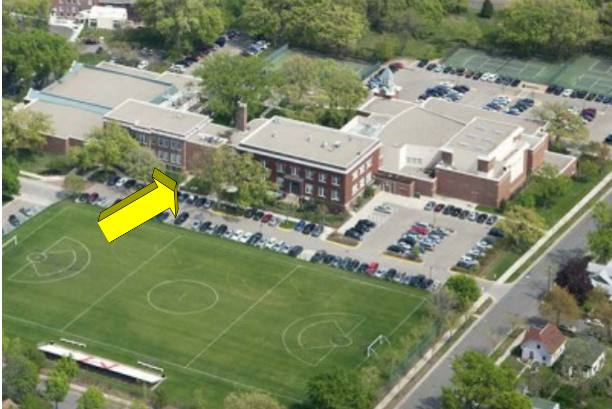
Figure 1. Aerial view, prior to the accident, of the North Campus of the Minnehaha Academy; yellow arrow indicates the area of the explosion. (Photo courtesy of minnehahaacademy.net)
