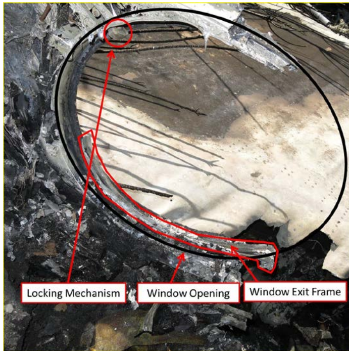
Photograph 23. Right side aft emergency overwing exit windows (outlined in black) depicting the locking mechanism, window opening and remaining window exit frame.
