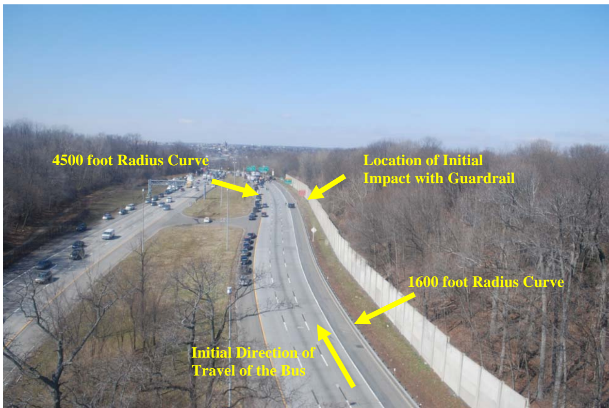
Figure 1 – Aerial view of roadway looking southbound.
