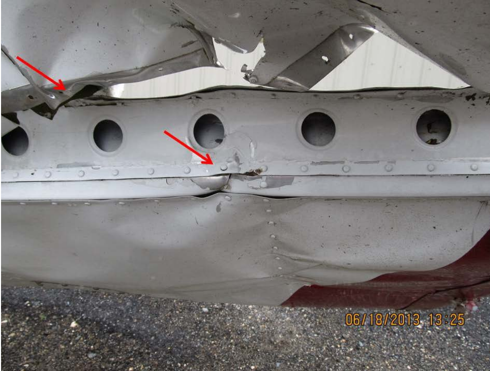
Photo 17 - The outboard section of the rear spar has compression damage on the top and bottom rear spar cap.
