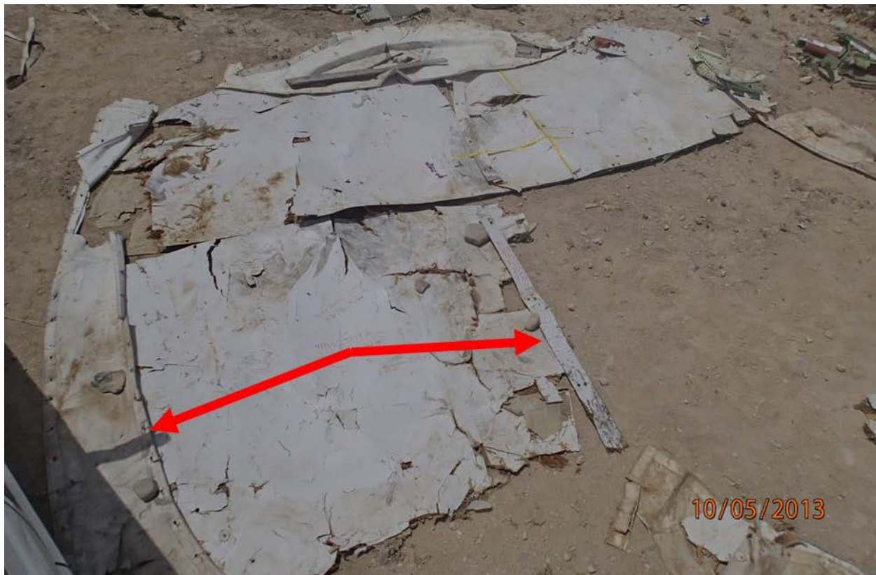
Figure 45 - Trapped APB Liner Material (1) & (2) reference Figures 39 & 40
