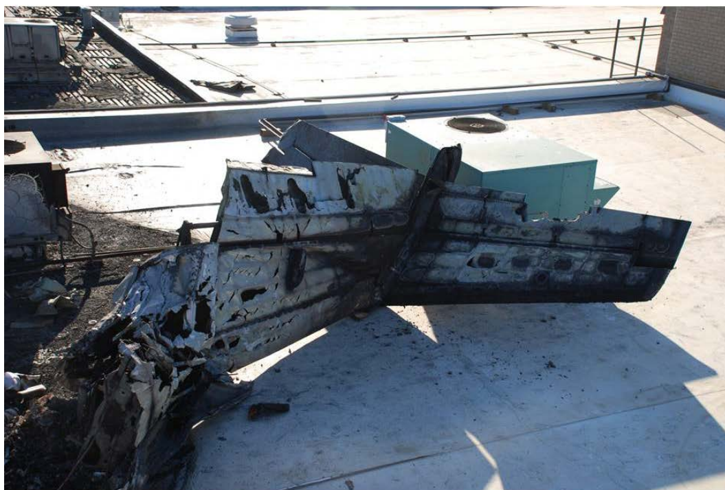
Photo 7 – Vertical and Horizontal surfaces on 2 nd roof level
