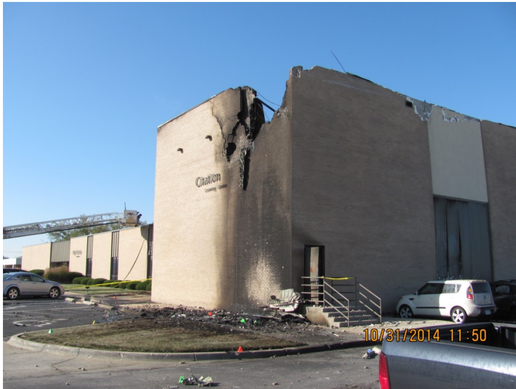
Photo 2 – Northeast corner of simulator bay
