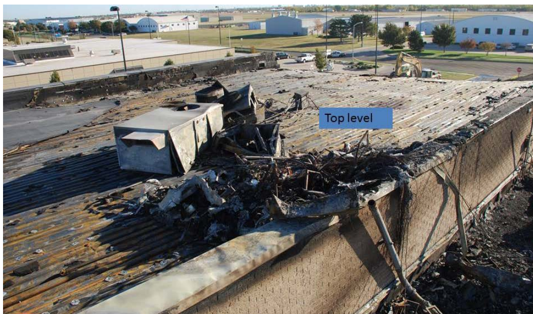
Photo 5 – Area of fuselage and instrument panel on top roof level. The initial impact area is at the top of the photo.
