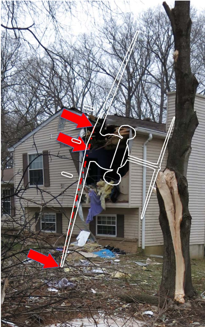
Figure 11. Aligning three points in path of left wing tip are the initial hole in the roof, the hole in the bedroom interior wall, and the hole in the yard. The dashed red line is along the wing leading edge and the airplane is shown only for rotational orientation. (The scale with respect to size is only correct for one point along the path toward the viewer.) At the bottom of the photo is a hole filled with water and the diameter of the hole is about that of the fuselage.
