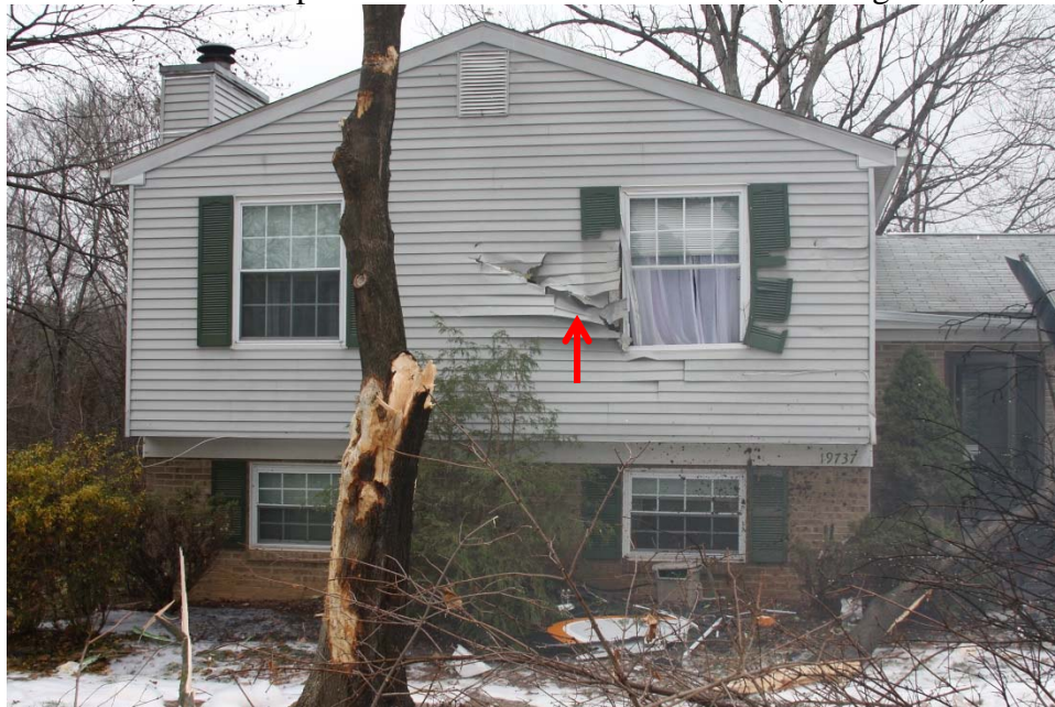
Figure 15. Exterior cut and damage to front of 10737 Drop Forge Lane at bedroom window. The airplane tail is at the right edge of the photo, partially blocking the front door. The arrow points to the carbon elevator fragment shown in the next photograph, from the trailing edge.
