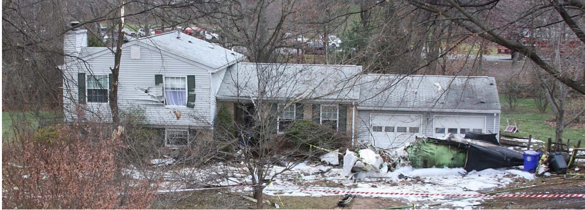
Figure 14. Overall view of 19737 Drop Forge Lane.
