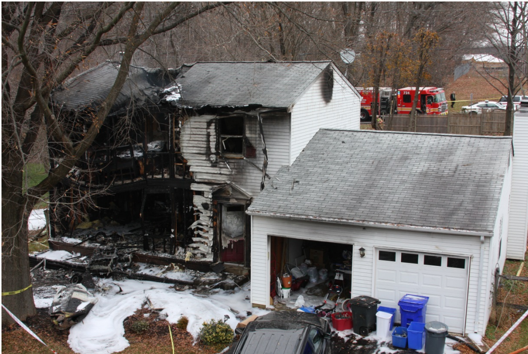
Figure 29. Overall view of 19733 Drop Forge Lane.
