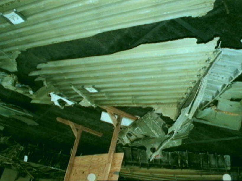
Structures 7 - V-5 Photo 2
