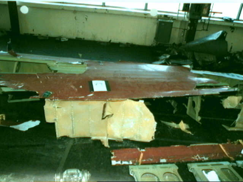
Structures 7 - V-4 Photo 1
