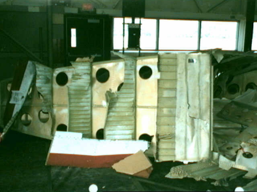
Structures 7 - V-2 Photo 3
