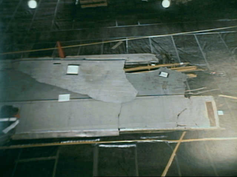
Structures 7 - RW-9 Photo 2
