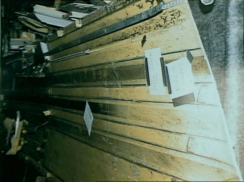
Structures 7 - RW-8 Photo 4
