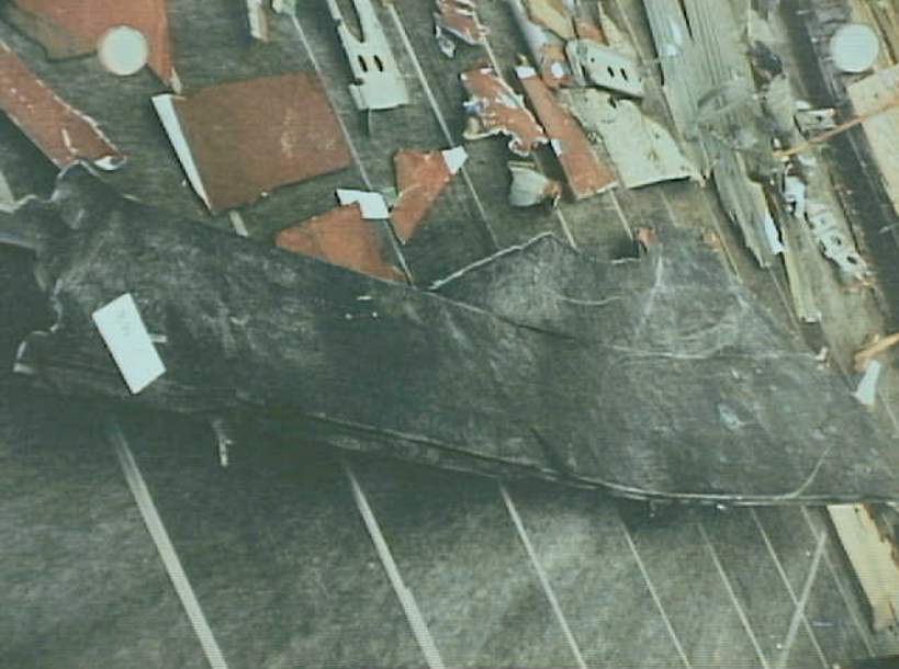
Structures 7 - RW-7 Photo 2
