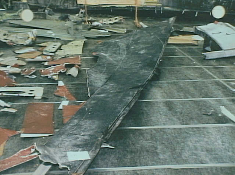
Structures 7 - RW-7 Photo 1
