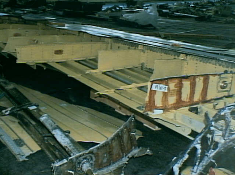
Structures 7 - RW-4 Photo 9
